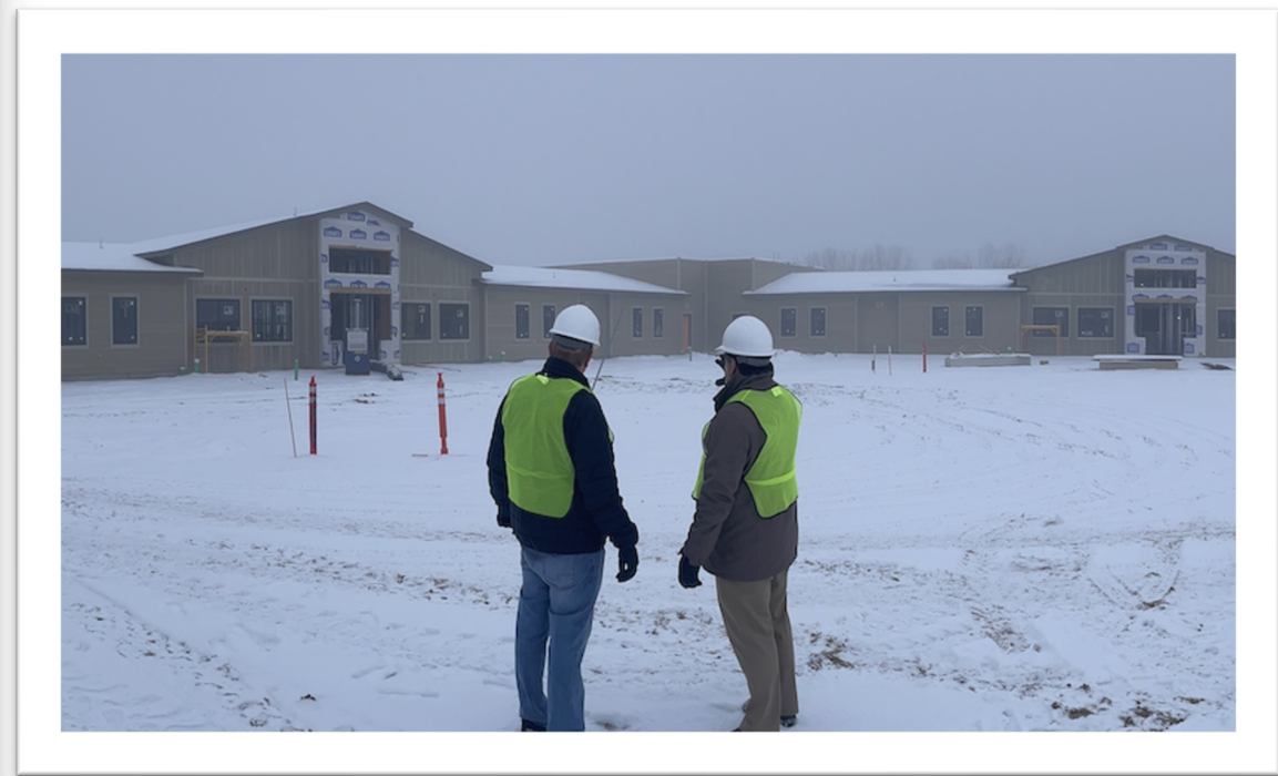
Image: New Charter School Construction, Middleton
